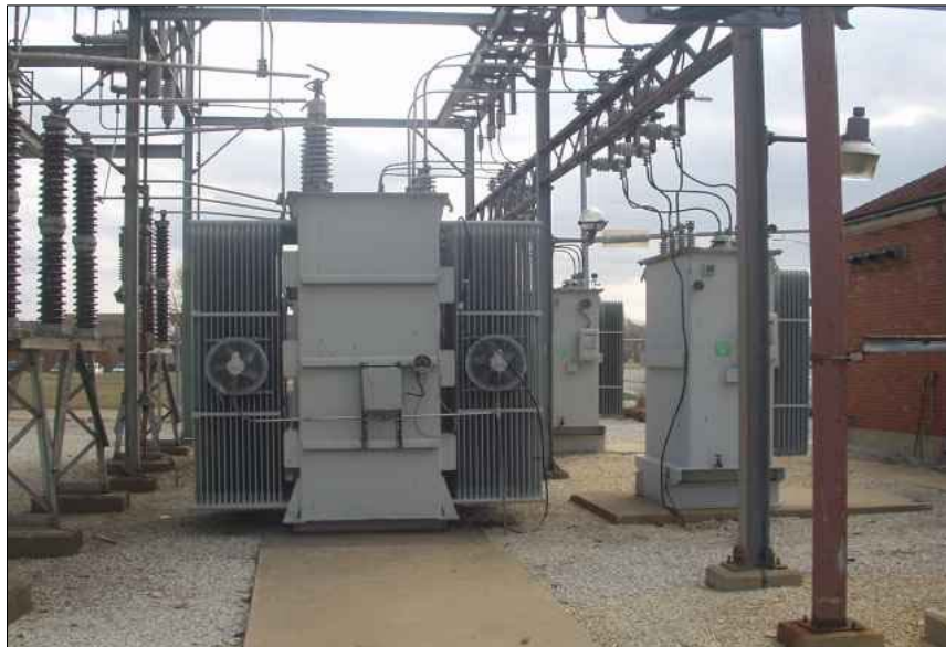
Oil Filled Transformer With Forced Air Cooling
