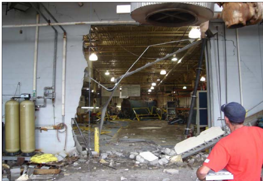
Hole In The Wall Created By Boiler Explosion
