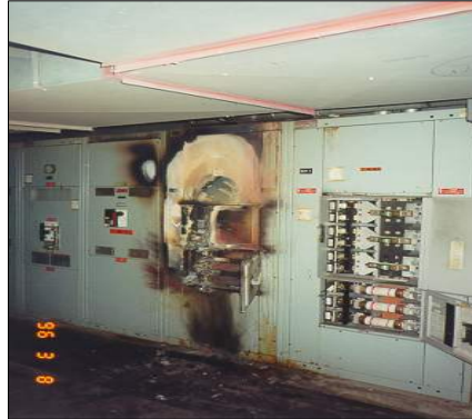
Electrical Switchgear after an arcing loss
