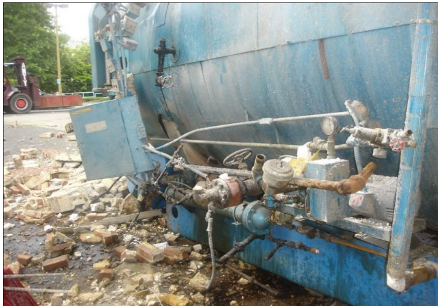
Substantial Damage To The Fire Tube Boiler
